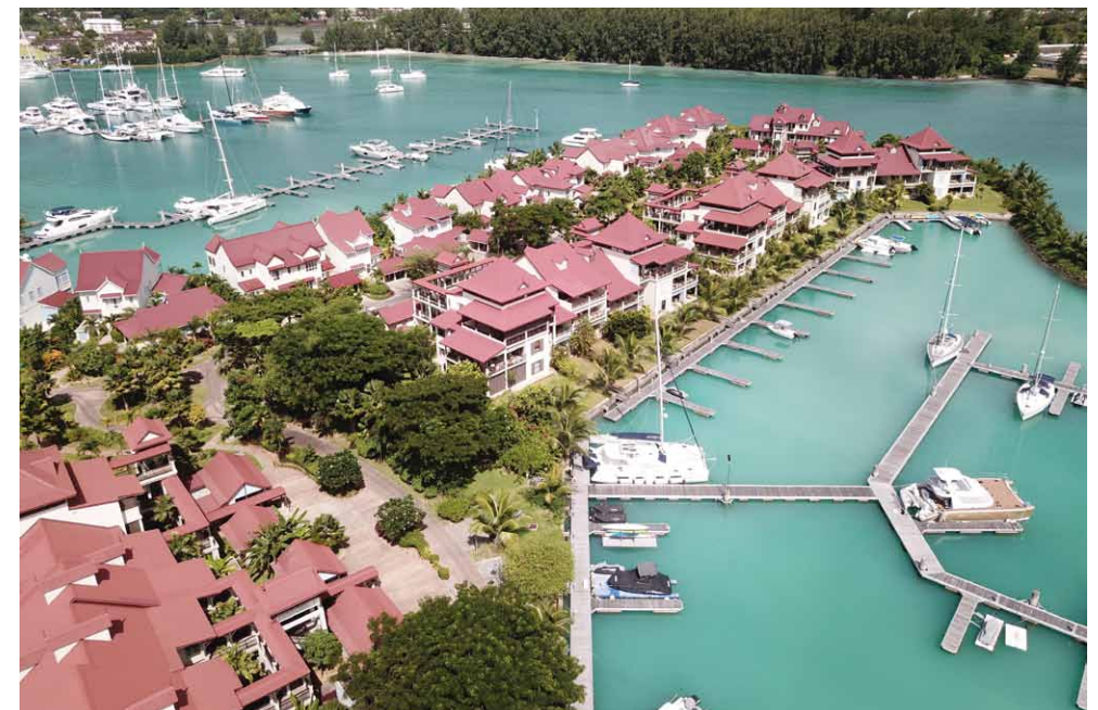
Aerial view of Eden Island Marina.
